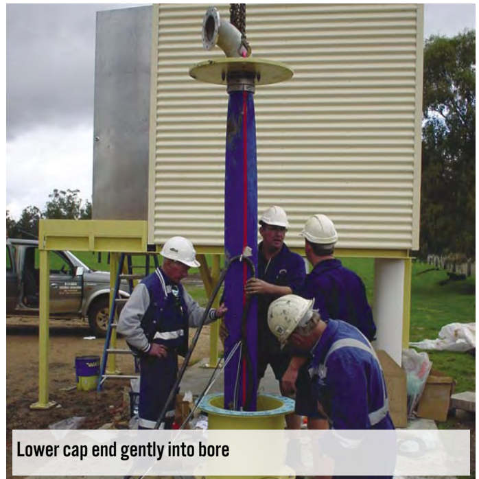
Clamp resting on casing holds weight of pump
