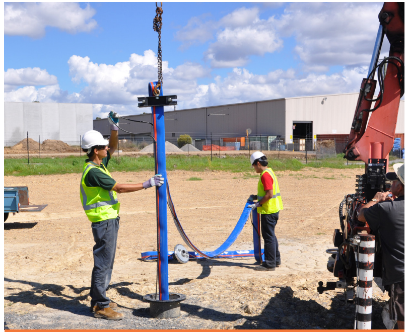
Lifting clamp for easy and safe Flexibore installation
